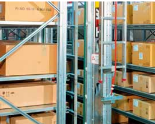
VMS for acceleration of storage processes
